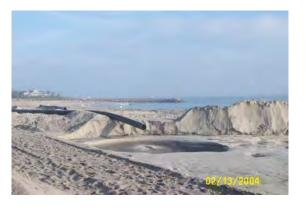
from the trap. To minimize the erosion problem occurring south of the south jetty, the University has recommended that a minimum of 60,000 cubic yards be pumped to the south beach on an average annual basis. Jupiter Inlet Sand Trap Dredging History
